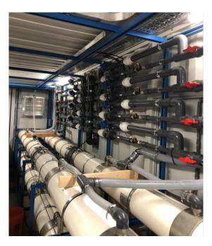
The customer was looking to standardize their proprietary pre-treatment for high salinity wastewater (120,000-130,000 ppm NaCl) and pair it with and liquid-solid separation step. The final goal was to create a containerized system that could be moved from site to site
